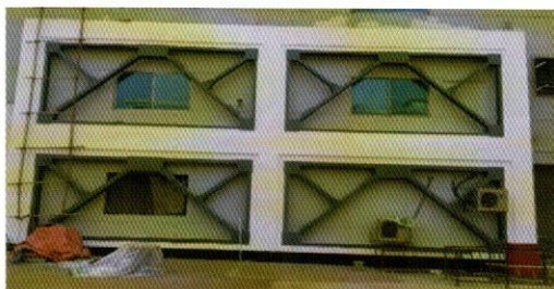
After Completion of Fixing Steel Frame Bracing
