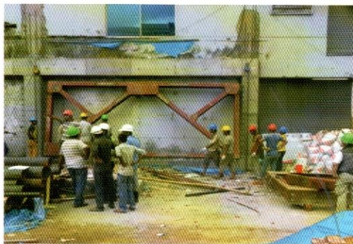
Installation of Steel Frame Bracing
