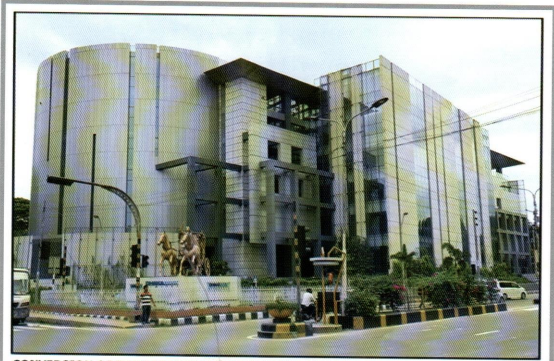
CONVERSION OF BANGABANDHU SHEIKH MUJIB MEDICAL UNIVERSITY (BSMMU) IN TO CENTRE OF EXCELLENCE PROJECT AT SHAHBAGH, DHAKA.
