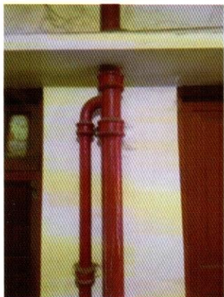
Figure1a. Upright-Wye' in the vent pipe system
