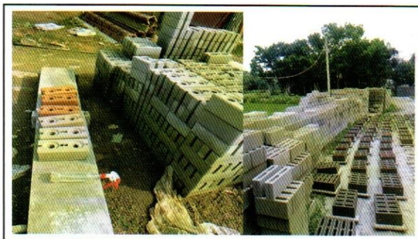
Fig 3: CSEB and Concrete Block produced at site
